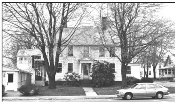
242 Main St - the Nathan Gillum House (History & Architecture Portland, 1980)
