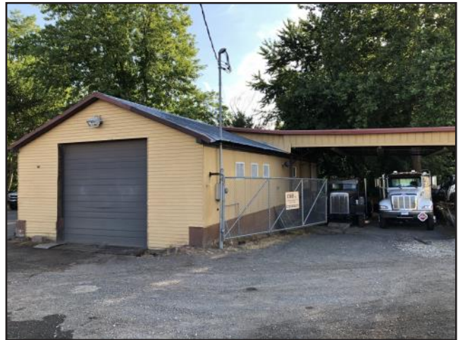
The CSB garage on Brownstone Avenue where all building and maintenance is performed.
