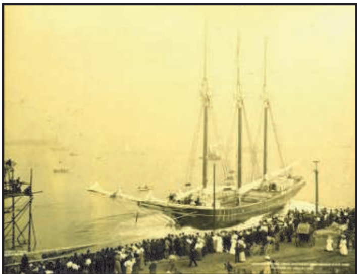
Launching of Schooner Frank Brainerd in Rockland, Maine, September 24, 1908.
