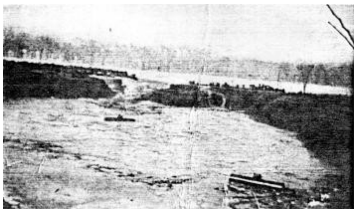
The quarry dike breaks. Note floating tank cars.
