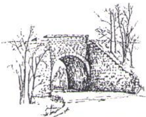
RAILROAD BRIDGE ON MIDDLE HADDAM ROAD
